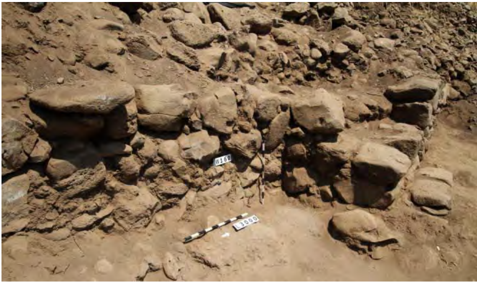
Figure 54. The projection off the city wall W160 marks a tower built into the city wall. Notice the two stones adjacent to the corner of that projection. This projection is echoed
