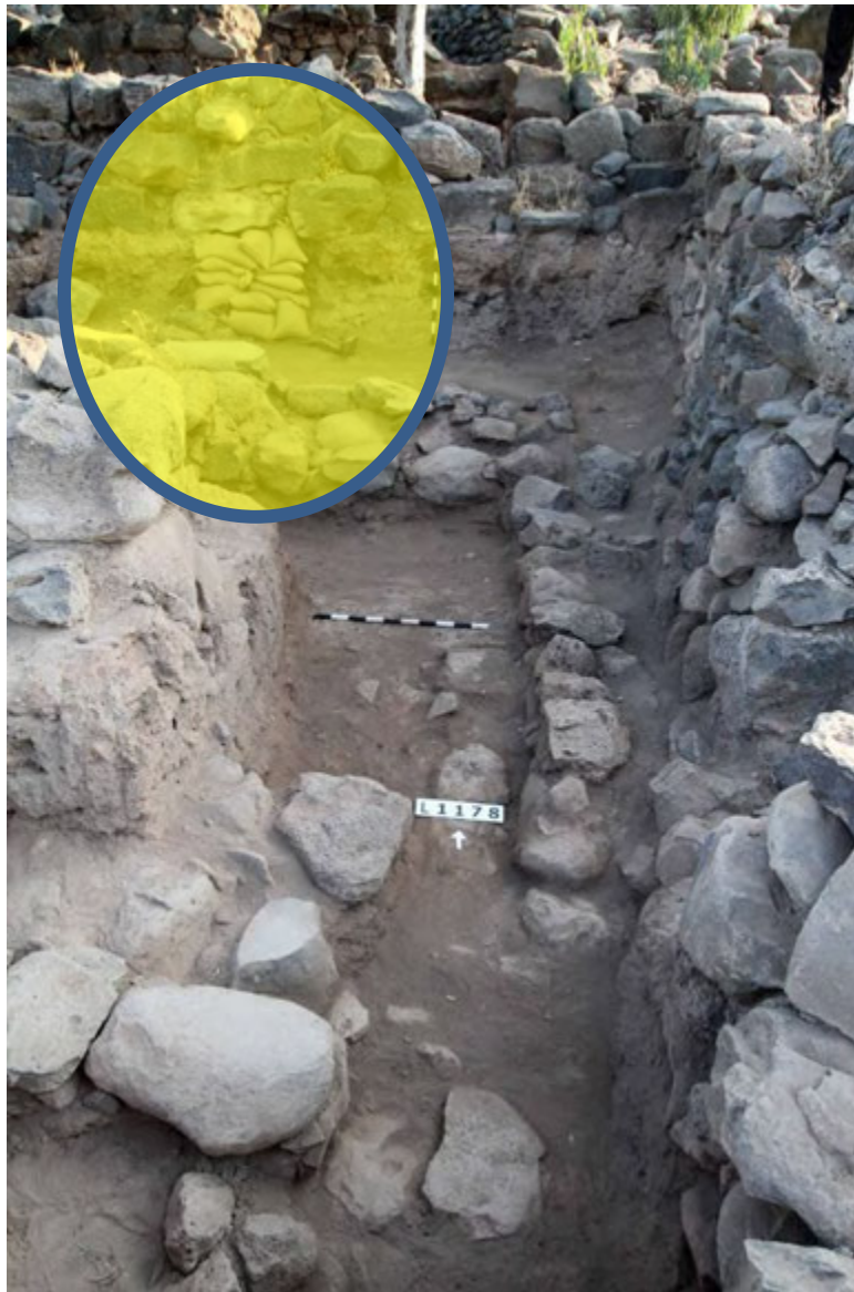
Figure 137, Conservation works has been done to support areas needed attention such as this one.
