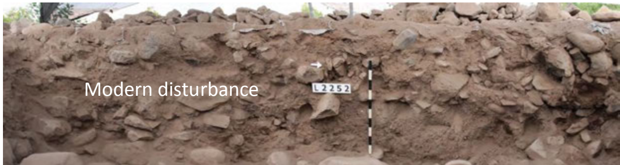
Figure 64, A section in area A West, looking west, showing 1.5 m of disturbed material.
