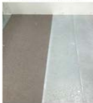
Compliant Cold Room
