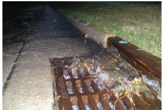
Figure 1. Stormwater runoff flowing into a storm drain. From here it flows directly to a nearby stream, river, or other surface water body.
