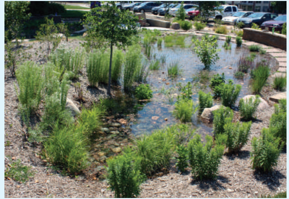
Figure 2. A bioretention garden after a rainstorm. Bioretention gardens capture and filter runoff and let it soak into the soil, usually within 24 to 48 hours.
