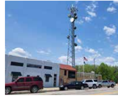
Ainsworth Cell Tower
