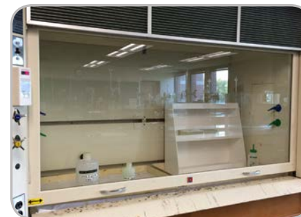
Figure 38: Another energy-saving opportunity is for campus users to appropriately shut fume hoods to minimize unnecessary ventilation
