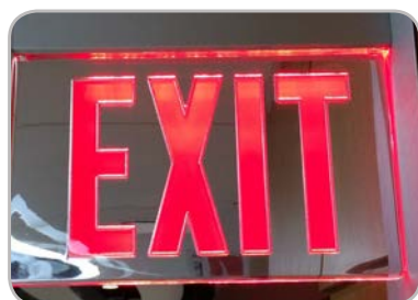
Figure 36: UNO should expect noticeable energy savings by replacing its older exit signs with newer ones that utilize LED technology.
