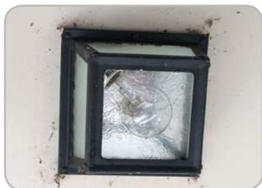
Figure 35: UNO should replace all incandescent bulbs, like this one at University Village, with CFLs or LEDs. The payback period for a CFL is typically less than 12 months while the payback period for a LED can range from 12 - 36 months.
